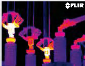
Thermal inspection of a high voltage installation.
